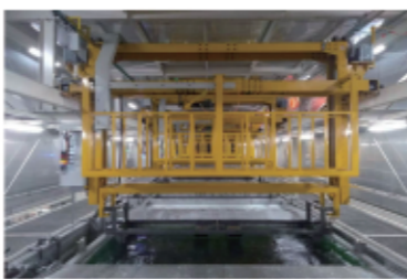
● 车架电泳线 Automotive chassis E-coating line
