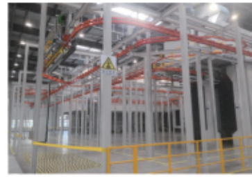
● 智能输送 Installation conveyor
