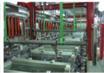
● 氧化/磷化设备 Oxygenation equipment Phosphorization equipment
